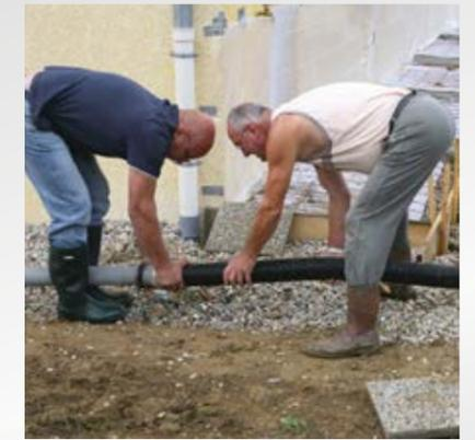
The delivery line is quickly laid and routed. A total of 45 m of delivery hoses and 45 m of delivery line are carried with the pump.
