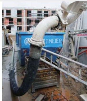
In closely-spaced housing developments, the 20-4 Sanima is a step ahead: With an extension line connected to one of the boom ends, concrete can be placed over distances that even the long 60 m booms can not span.
