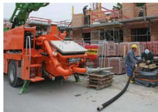
The 20-4 Sanima as pure hose pump: With the hinged elbow rotated by 180°, reduction couplings for DN 65 delivery hoses can be connected. Here, the 20-4 Sanima is used in restricted space to pump concrete into cellars through more than 80 m of delivery line.
